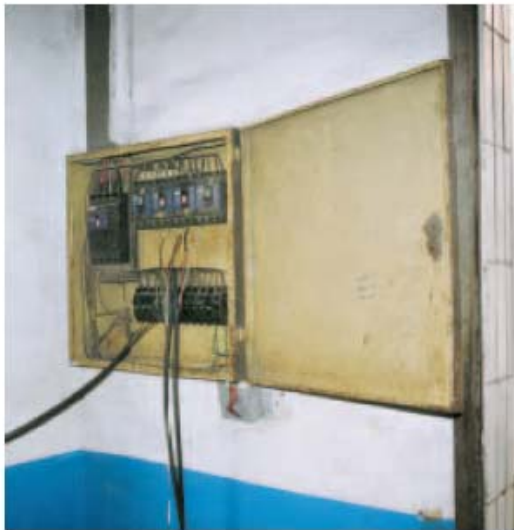
typical electric hazards
