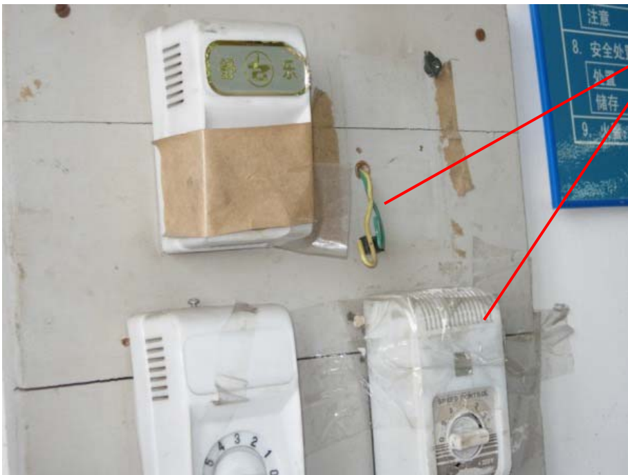
Figure 11.14 – Poor Maintenance of Machine Switches
