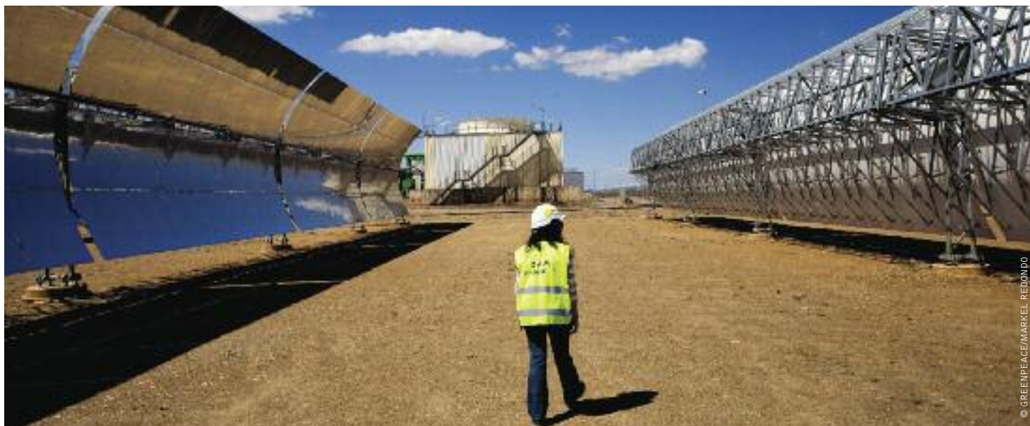
image A WORKER SURVEYS THE EQUIPMENT AT ANDASOL 1 SOLAR POWER STATION, WHICH IS EUROPE'S FIRST COMMERCIAL PARABOLIC TROUGH SOLAR POWER PLANT. ANDASOL 1 WILL SUPPLY UP TO 200,000 PEOPLE WITH CLIMATE-FRIENDLY ELECTRICITY AND SAVE ABOUT 149,000 TONS OF CARBON DIOXIDE PER YEAR COMPARED WITH A MODERN COAL POWER PLANT.
