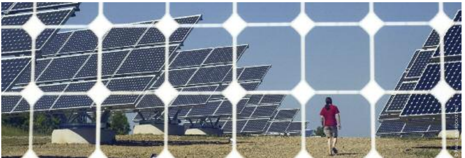
image SOLON AG PHOTOVOLTAICS FACILITY IN ARNSTEIN OPERATING 1500 HORIZONTAL AND VERTICAL SOLAR "MOVERS". LARGEST TRACKING SOLAR FACILITY IN THE WORLD. EACH "MOVER" CAN BE BROUGHT AS A PRIVATE INVESTMENT FROM THE S.A.G. SOLARSTROM AG.
