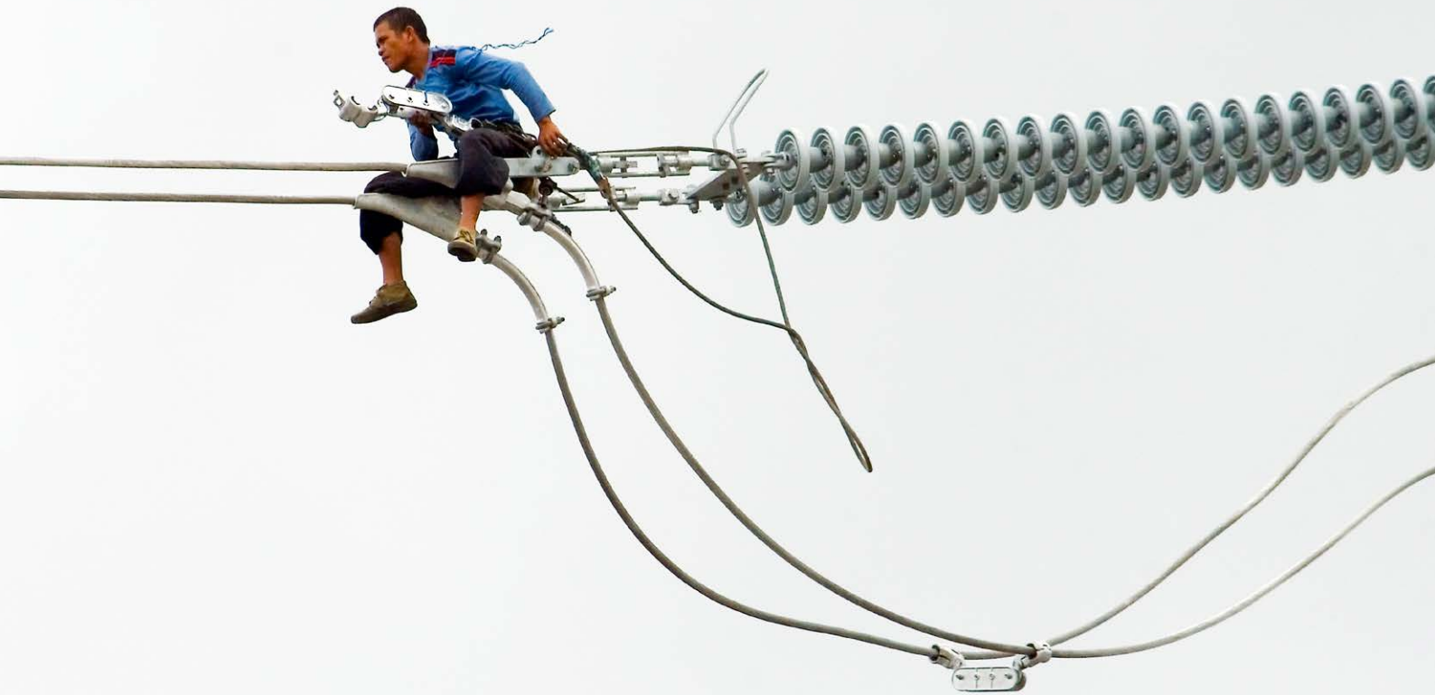
A worker installs a new electric cable atop a pylon in Philippines. © Bobot Go/ILO
